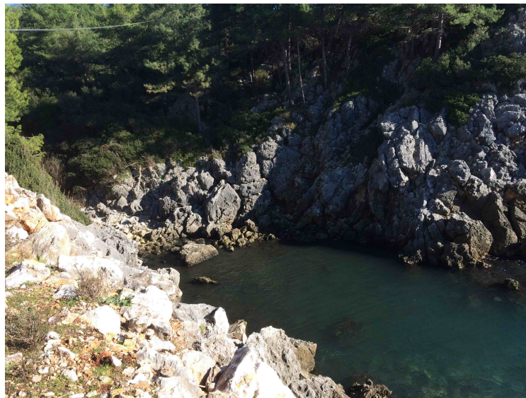
Figure 4-16: Overflow of pumped wastewater into a bay (Siemers 2016)
