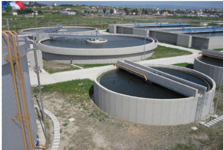
New Wastewater Treatment Plant in Durres
