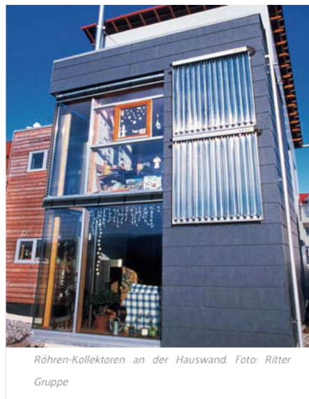
Figure 4-10: Pipe solar collector on the wall as vertical installation (Ritter 2017)
